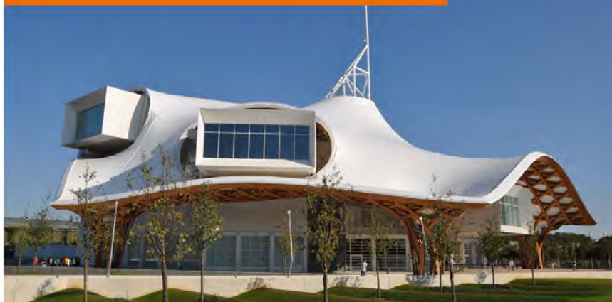
Centre Pompidou-Metz, Shigeru Ban Architects, 2010, Foto © archiv Hermanna Blumera
